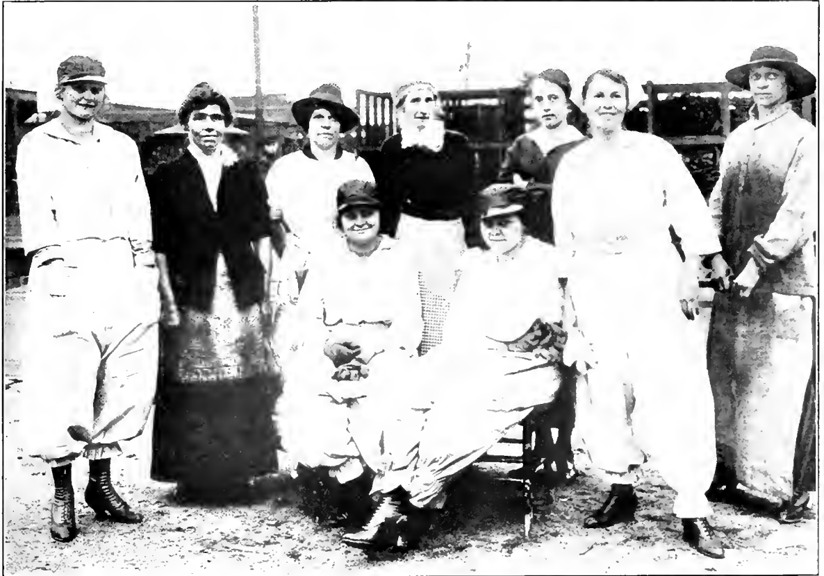
Women Employed in the Baltimore & Ohio Shops at Lorain, Ohio
